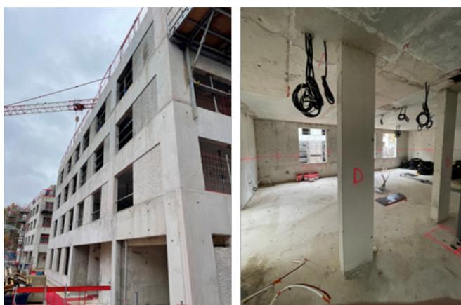
Fig. 1, Construction site I3F (France, 2022). All concrete on the photo is based on GGBS activated by Na<sub>2</sub>CO<sub>3</sub>
