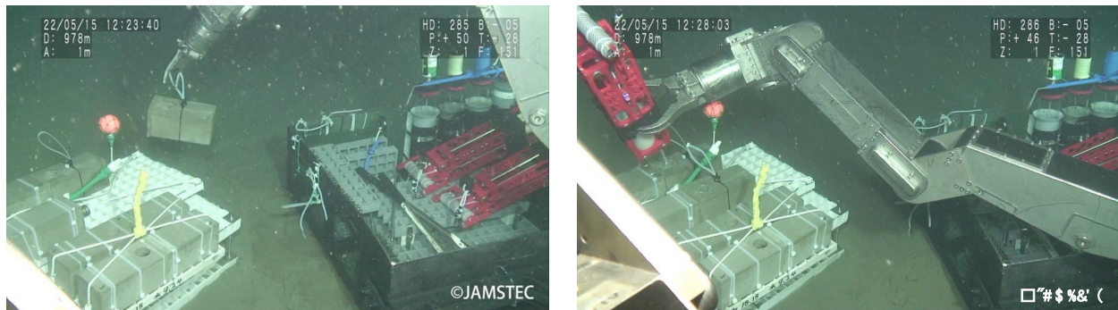
Fig. 3 Connecting of precast mortar members on the seafloor with a depth of 980 m by using the deep-submergence research vehicle Shinkai 6500 (left) and discharging of the mortar and activator conducted by manipulators (right). These photos were provided by Japan Agency for Marine-Earth Science and Technology (JAMSTEC).
