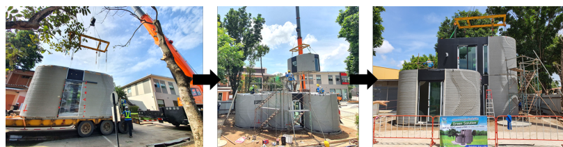
Figure 3: On-site Installation and Finishing
