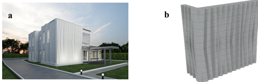
Figure 1: a. Final design of "SCG Health center" building b. The texture of 2-storey non-load bearing 3DP panel
