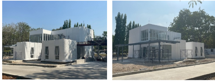
Figure 6: The 3D printed 2-story building
