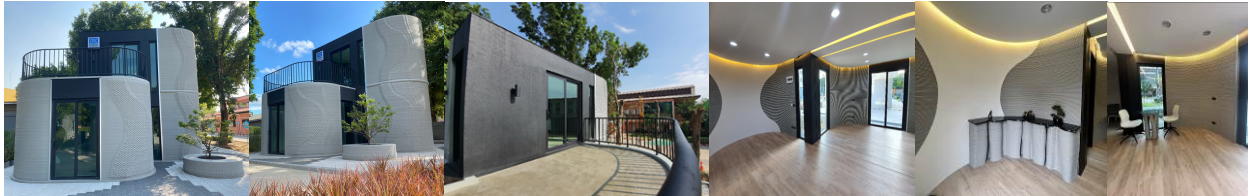
Figure 5: The exterior and interior of the building
