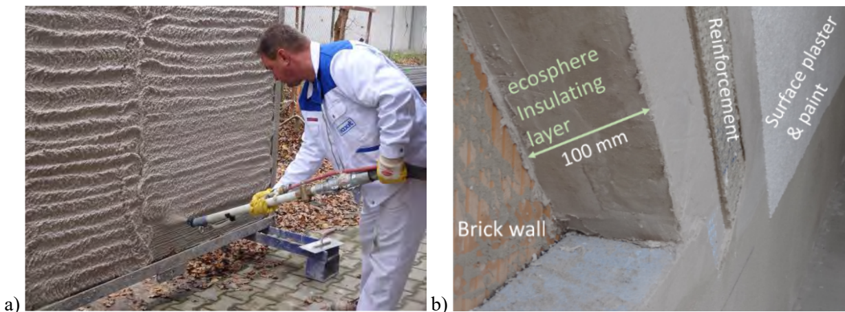
Figure 2. The insulating Ecosphere plaster: a) application of the plaster by spraying to a brick wall, b) cross-section after spraying with addition of a fibre-based reinforcement and surface plaster layer.
