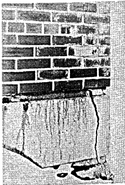
Figure 3: Expansion of walls with resultant rupture of concrete foundation.
