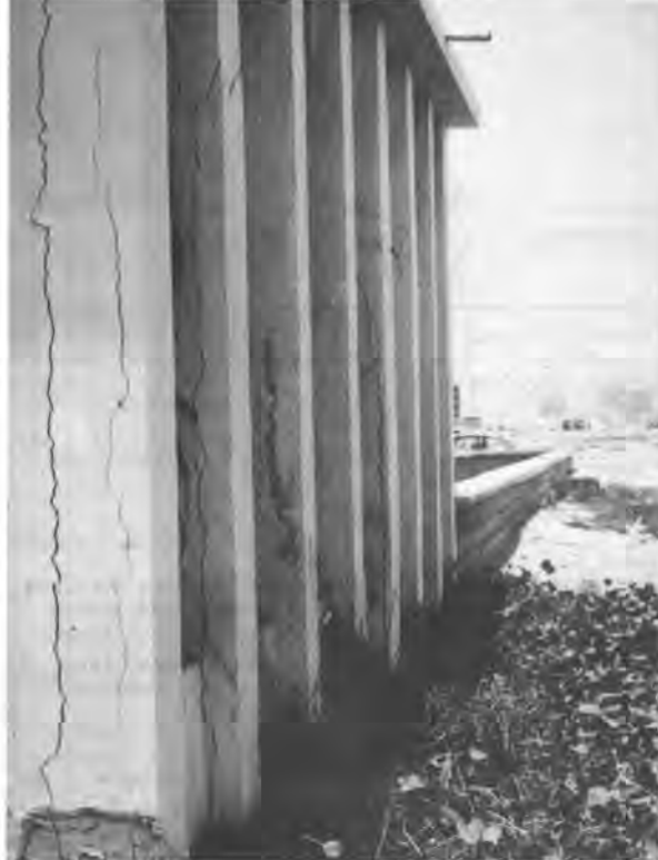
FIGURE 5 Concrete structure in a Middle East country. The concrete is thoroughly cracked due to severe corrosion of the reinforcement bars with expansive forces developed during the formation of corrosion-products. The corrosion is probably enhanced by capillary suction of salts from the groundwater, and definitely by the temperature-conditioned acceleration of all the involved physico/chemical processes.
